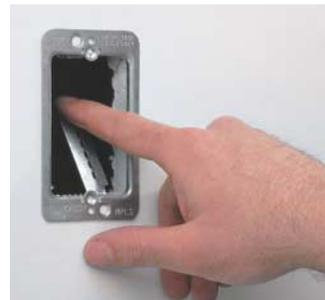
**Low-voltage mounting bracket:** For installing wall plates. Cut a hole in the drywall, bend the metal tabs behind the wall, then lock the tabs in place with screws. Then attach the wall plate to the bracket.
