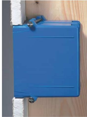
*If you're using half-inch dry-wall, install your J-boxes so that they protrude a hair less than half an inch from the front of your studs. When the walls go up, the boxes will be positioned perfectly.*
